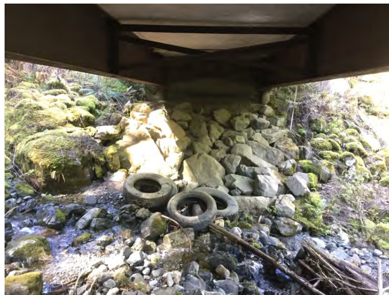
Left Bank Abutment when facing downstream
