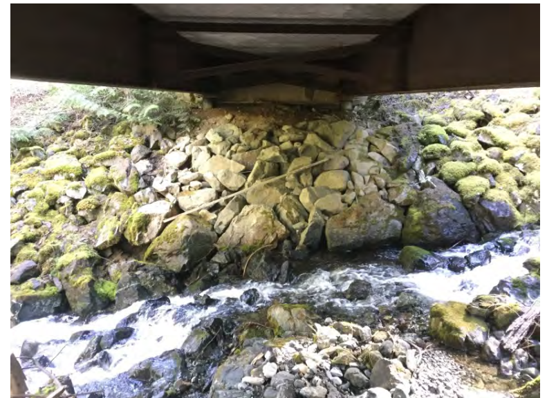
Right Bank Abutment when facing downstream
